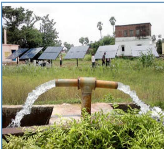
The photovoltaic pumps have many advantages including they operate on freely available sunlight and therefore incur no fuel or electrical costs. They are also environmentally friendly, reliable and have a long working life [1]. The advantage of using solar energy for pumping the water is that major quantities of water are required during day time and that too during time when the sun is on top of our head, and during these times the PV panels produce maximum energy and hence the water quantity.
