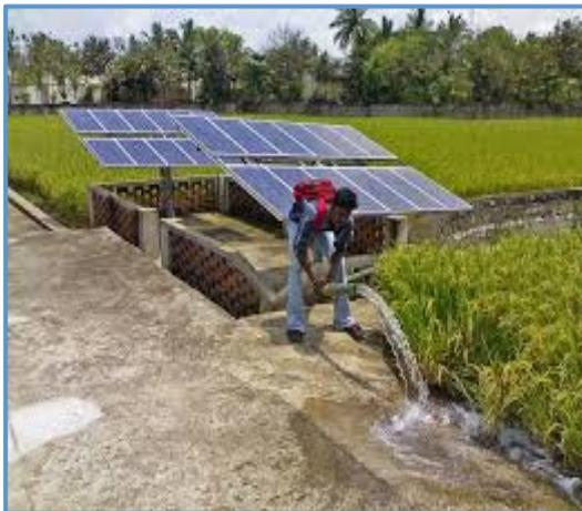
As always, each component causes a loss (photovoltaic modules 11%; motor-pump unit, cables and controls 45%). Therefore the actual hydraulic output, ignoring pipe losses will be about 5% of the power of the sun arriving through the window of the array. Pipe losses may be another 0.5% of the total input, giving at best an overall efficiency of 4.5%. Figure 7 illustrates the power flow through a typical photovoltaic pumping system
